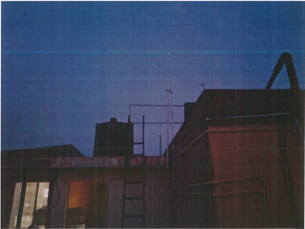
Water distribution system in the buildings of NSU
