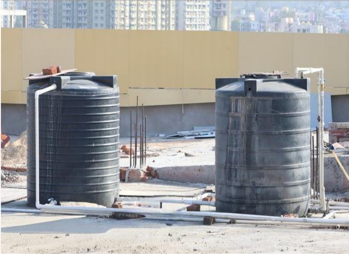
Water tanks in Chandrasekhar block
