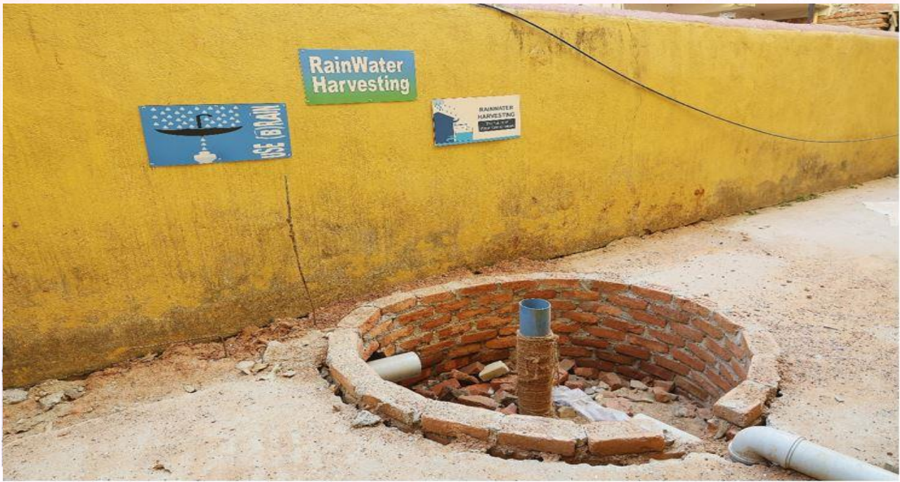
Rain Water Harvesting in the campus of NSU
