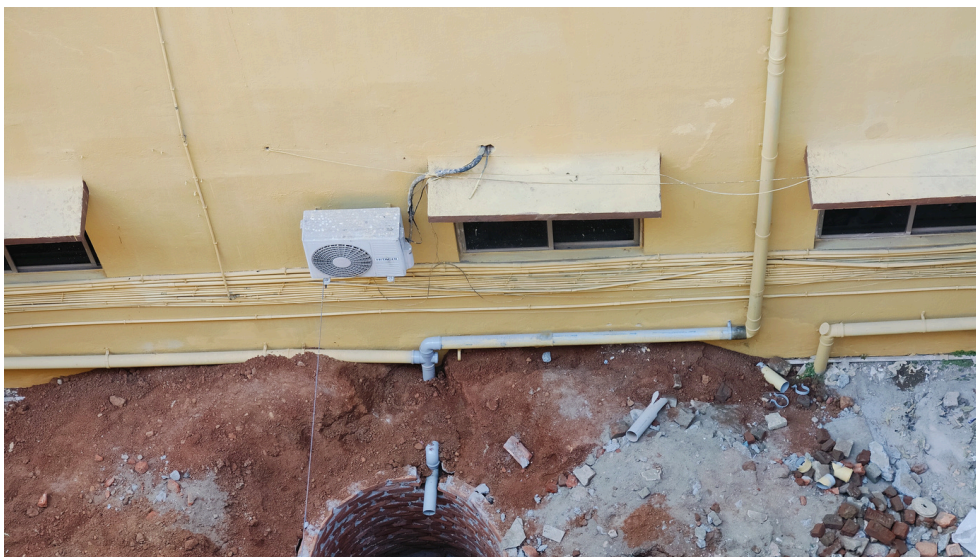
RAINWATER HARVESTING SYSTEM WITH FILTER, DOWNPIPES AND WATER COLLECTION CIRCUITS AT NETAJI SUBHAS UNIVERSITY
