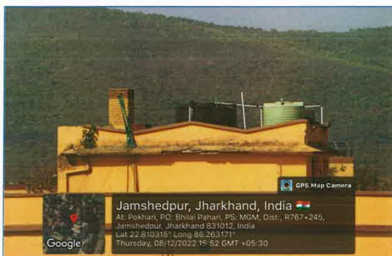
Water Tank: Shaheed Sukhdev Block
