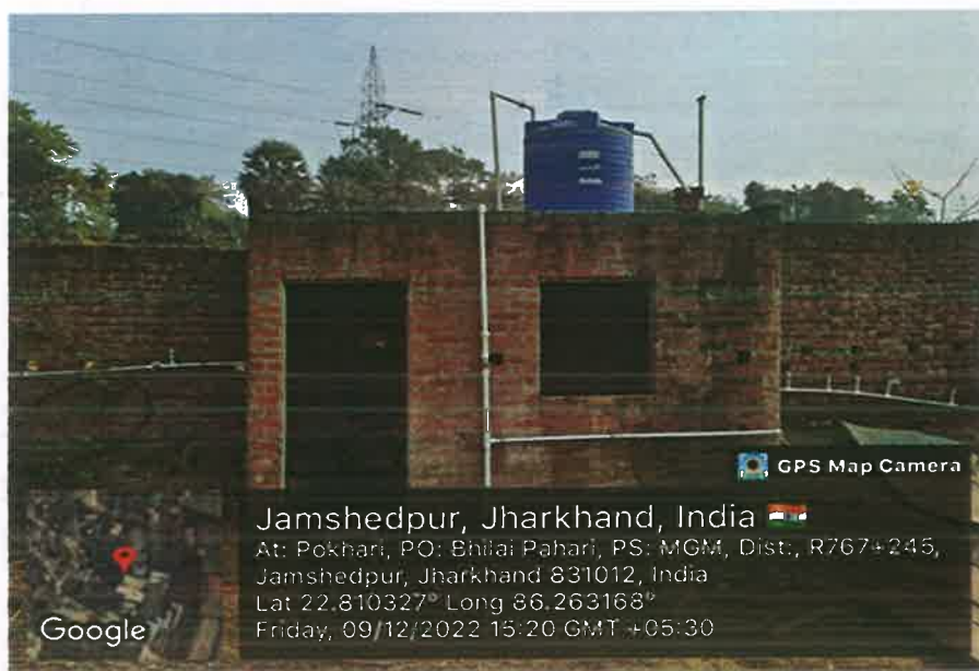
Waste water recycling center
