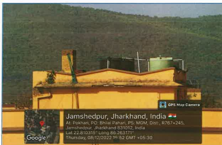
Water Tank: Shaheed Sukhdev Block
