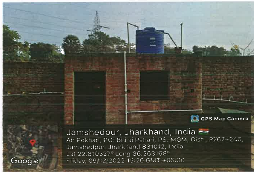
Waste water recycling center
