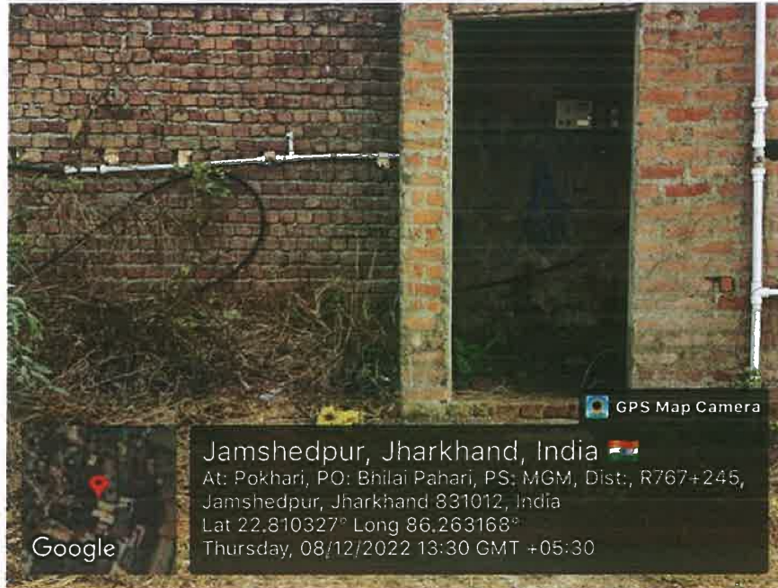
Waste water recycling center
